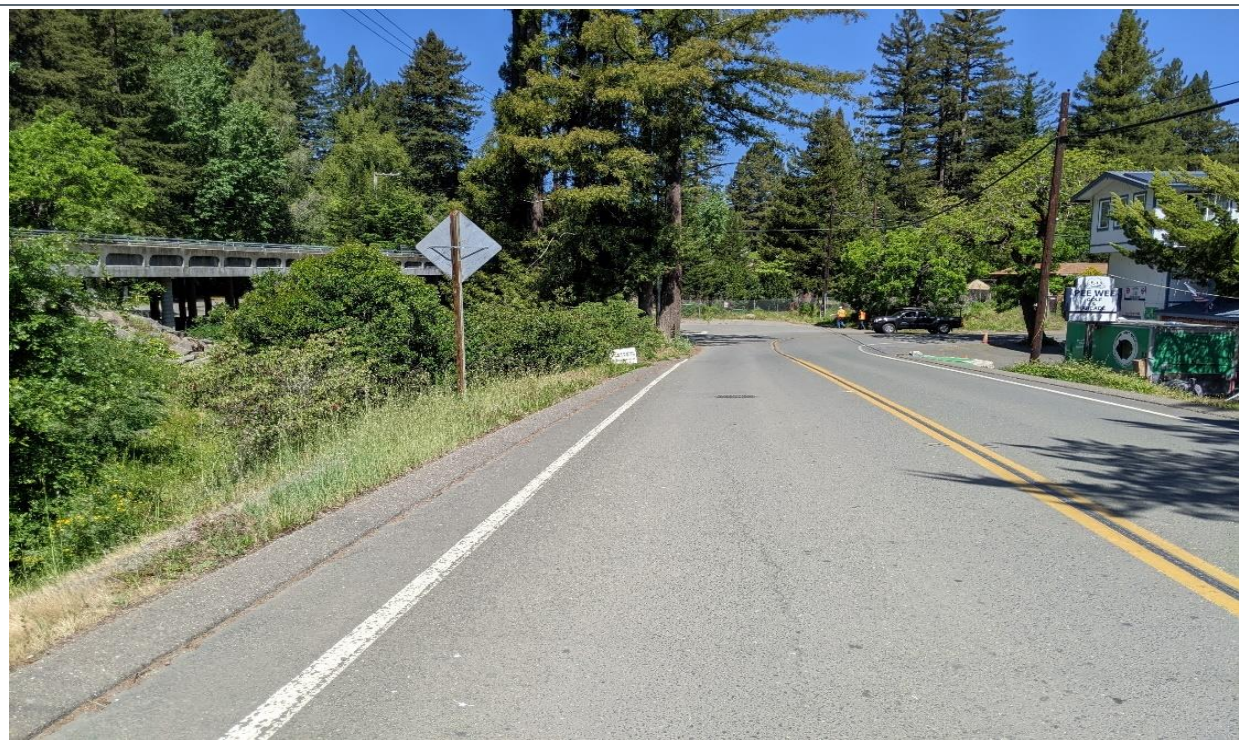
Photo 2 Looking northwest along Drake Road at the location of existing Segment 1 of the Beanwood Force Main and existing road conditions.
