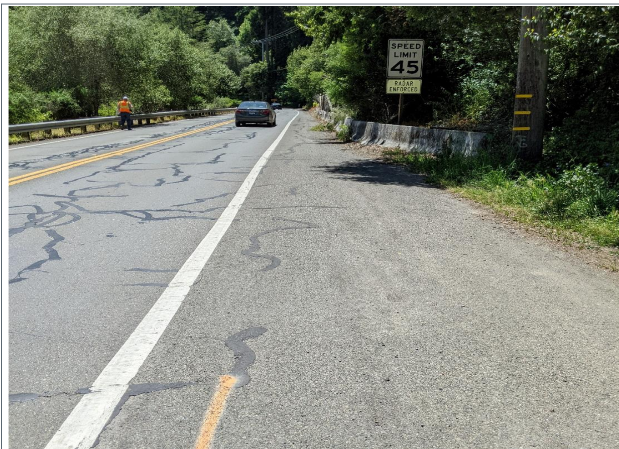
Photo 5 Looking southeast along Highway 116 at the location of the Segment 2 pipeline alignment.
