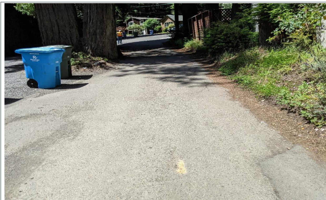
Photo 4 Facing northwest towards Highway 116 on Riverside Drive showing redwood tree obstructions.
